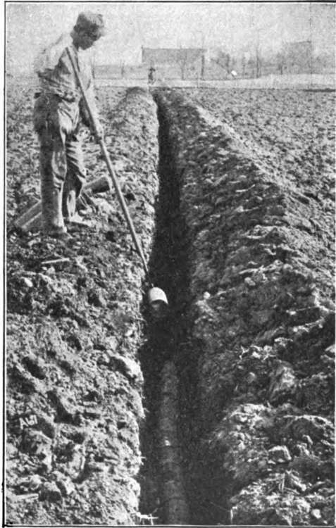
FIG. 267. — Tiling Level Lands, Illinois.
